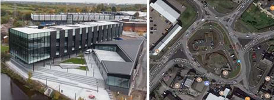
Figure 41: New Barons Quay Development (Left) and New Leicester Street Roundabout (Right)
